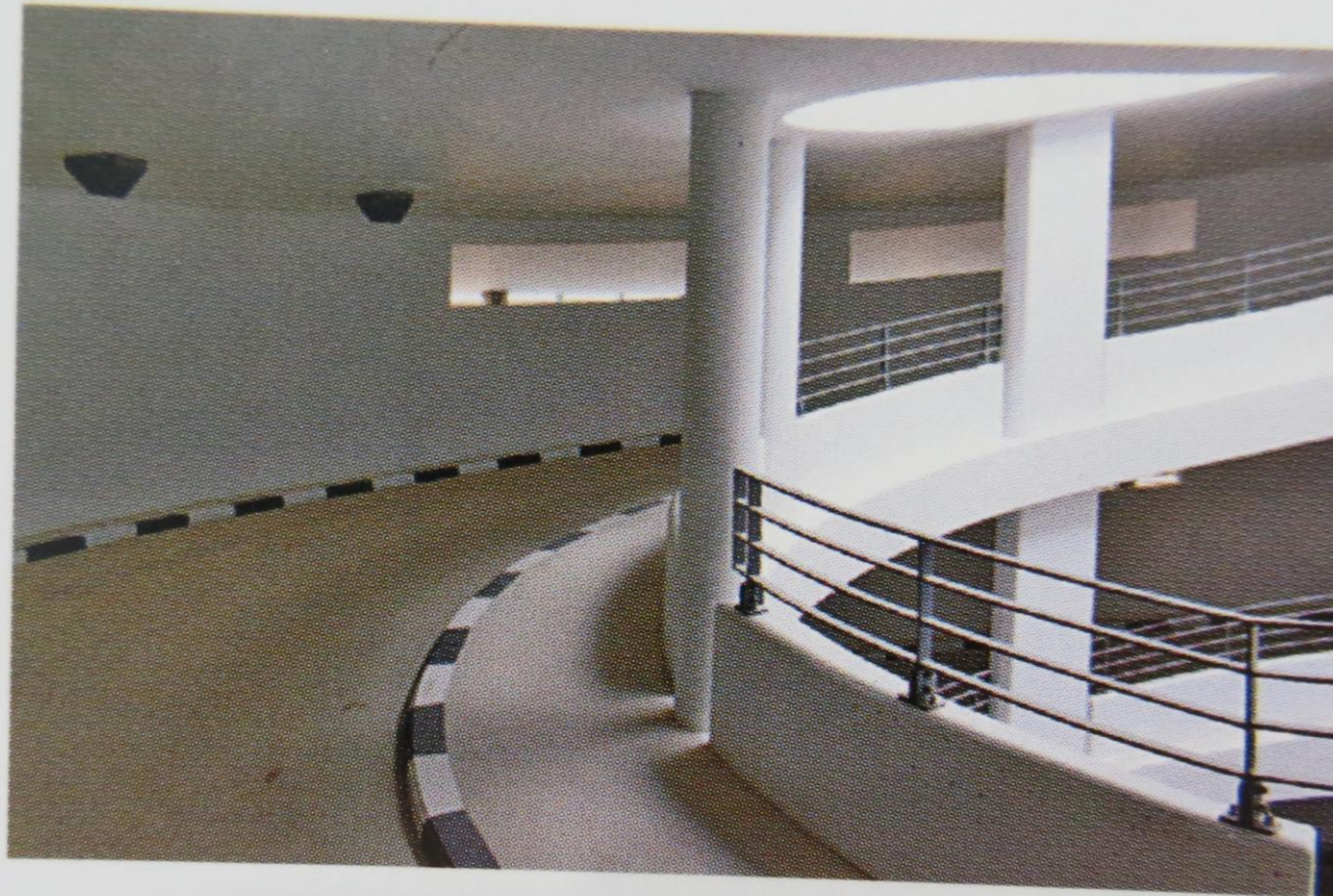
Image 109: EAR 05-compliant spiral ramp with all the required safety features ( Alter Steinweg, Münster )
