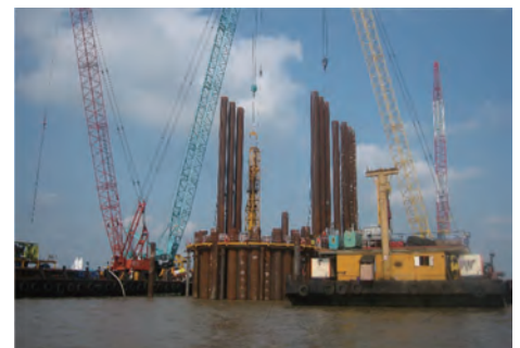
Photo 3 SPSP installation
