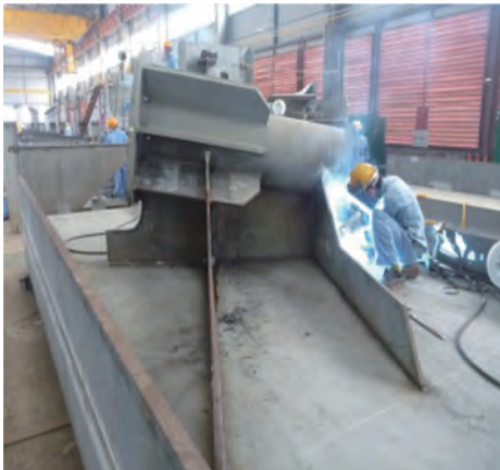
Photo 4 Steel fabrication works
