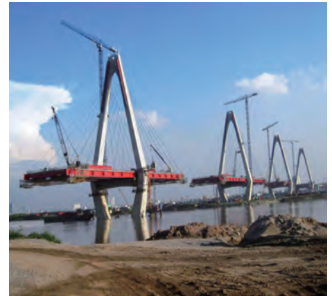
Photo 2 View of construction by cantilever erection
