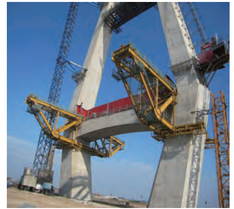
Photo 1 View of construction by inclined bent
