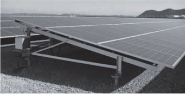
Photo 3 Solar panel framing
