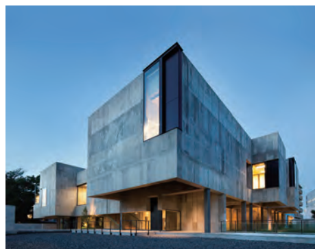
Photo 4 No. 1 Building of Toho Gakuen Chofu Campus
