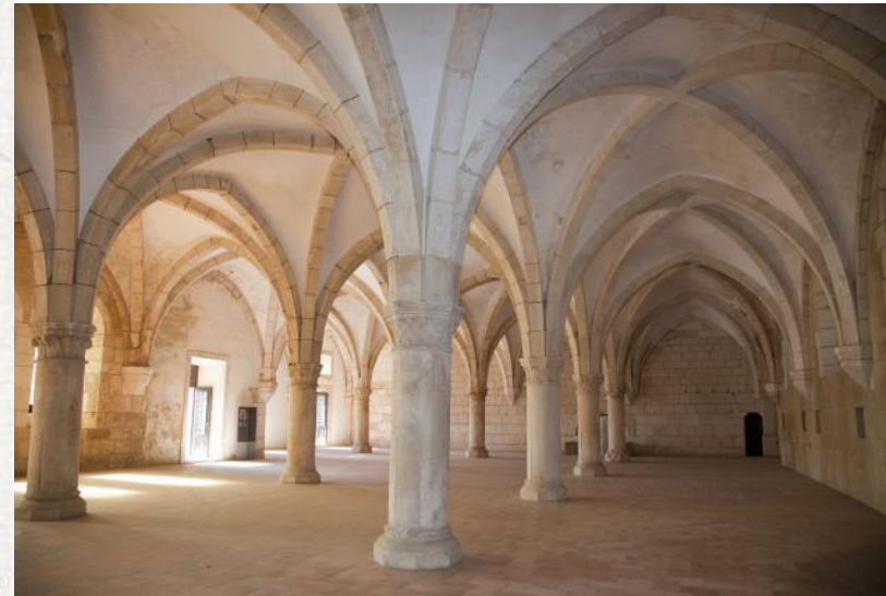
1, Gothic groined vault. 2, Spherical or domical vault.
