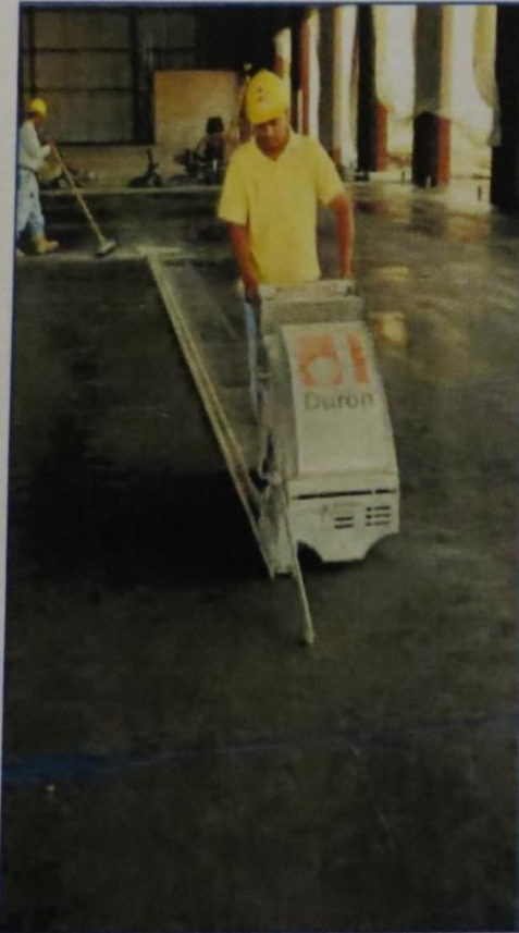
Fig. 11-27. Contraction joints provide for horizontal movement in the plane of a slab or wall and induce controlled cracking caused by drying and thermal shrinkage.
